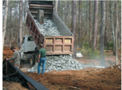
Figure 3 - Road construction introduces off-site materials which may contain invasives.
