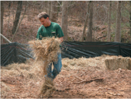
Figure 19 - Applying mulch for soil stabilization
